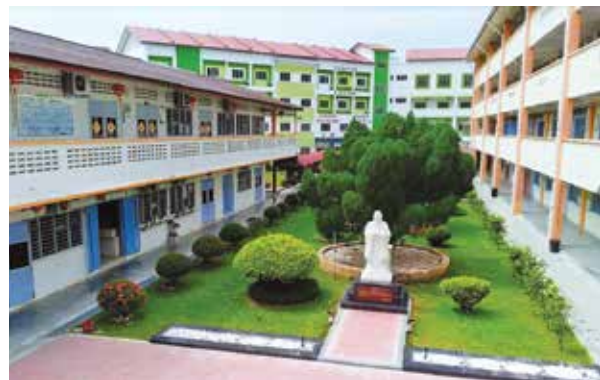
CM contributed RM5,000 to Sekolah Menengah San Min (Suwa) in May 2024 to support its building extension project.
